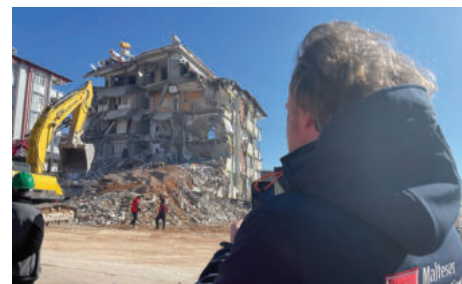
Oliver Hochedez on the ground surveying the extensive damage in the wake of the earthquakes in Türkiye and Syria in March 2023.
